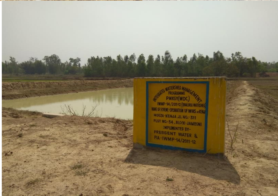
Construction of Water harvesting structure at Dakai watershed
