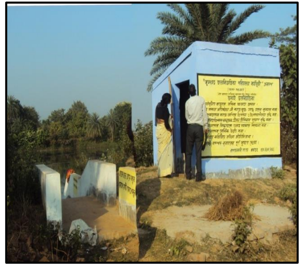
Bathing Ghat and cloth changing room under Entry Point Activity at Simulpal village
