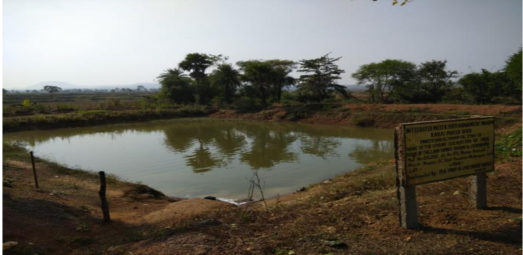
Views of Various Water Harvesting Structures at Different Villages of Dakai watershed
